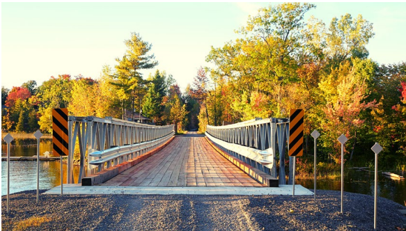
Trail of Two Lakes: Pedestrian Bridge Crossing Moira Lake (Kramp Crossing)
