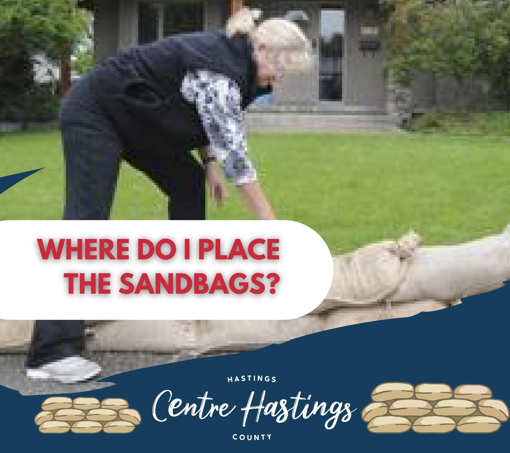
Build a small sandbag wall across external doorways. This includes sliding doors and garage roller doors. The height of the sandbag wall will depend on the expected height of the floodwater; however, it is generally around two sandbag rows high.
